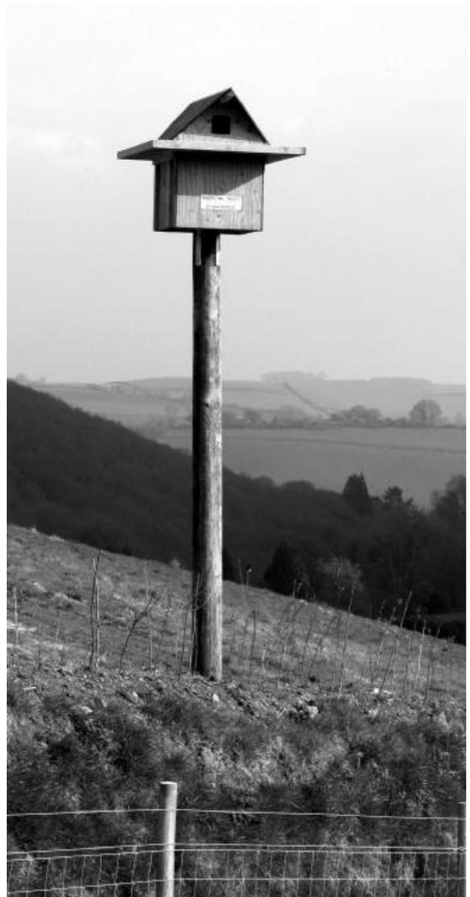
waterproof so the roof sheets should also be treated with Creosote or some other water-resistant preservative. The apex should be covered with a strip of aluminium or copper. The front, back and sides **MUST** overhang the floor of the box and as an extra precaution a large drainage hole (20mm -  $\frac{3}{4}$ " - diameter) should be drilled in each corner of the floor of the box.
